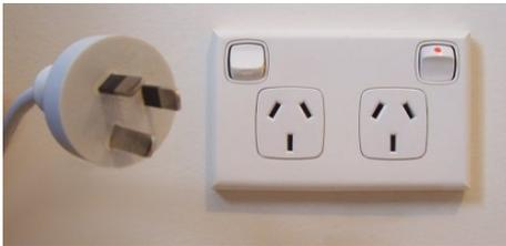
The standard voltage for electrical items in Australia is 240V. Electric plugs have three flat pins one of which is an earth pin. You may need to buy an adaptor or have the plugs changed when you arrive.
